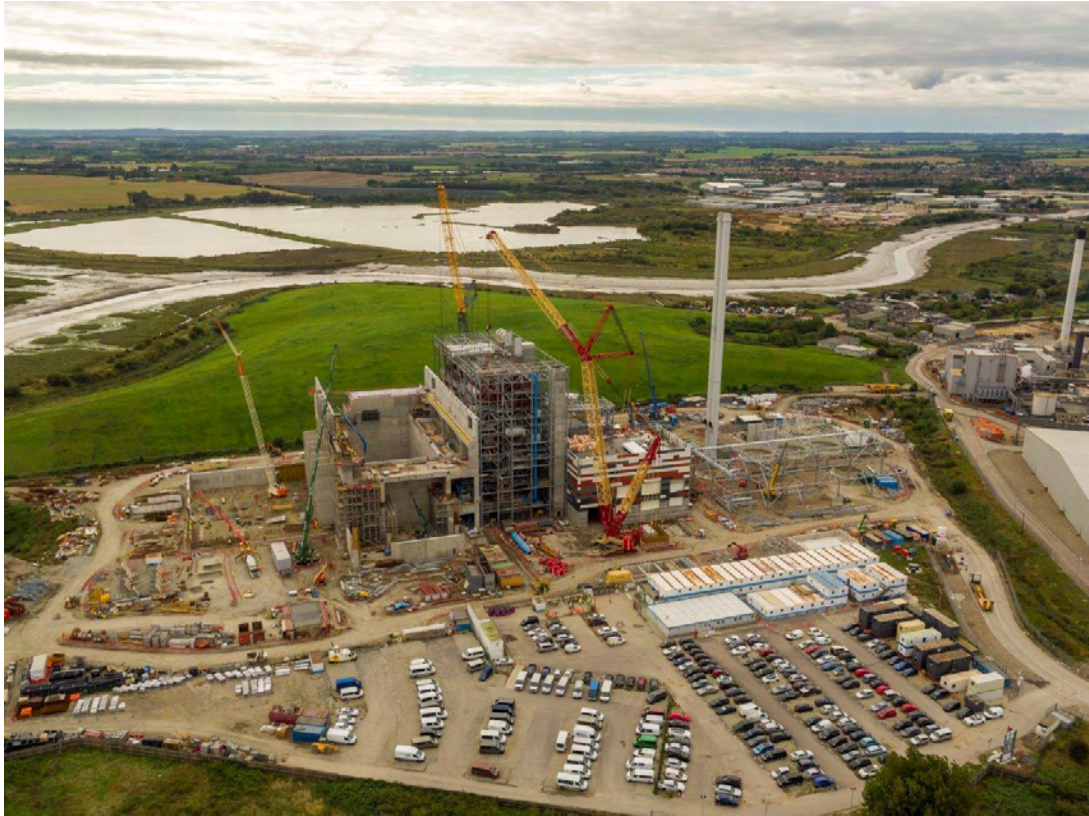
K3 – Construction progress at October 2018
